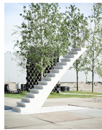
Figure 1.3: Staircase created with printed formwork
