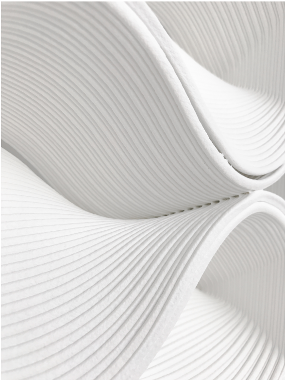
Figure 2.23: Close-up of a joint of the full-print façade. The intralayer bonds within the joint are clearly visible.
