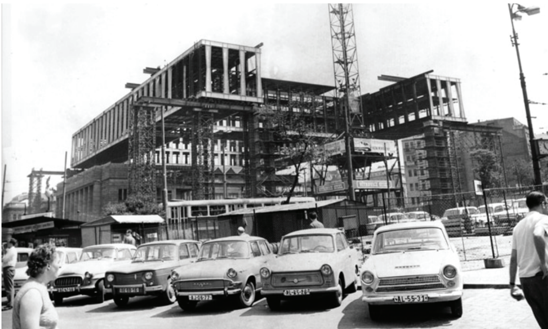
(Lifting of the Vierendeel trusses, 1969 (Marečková, 2013))
