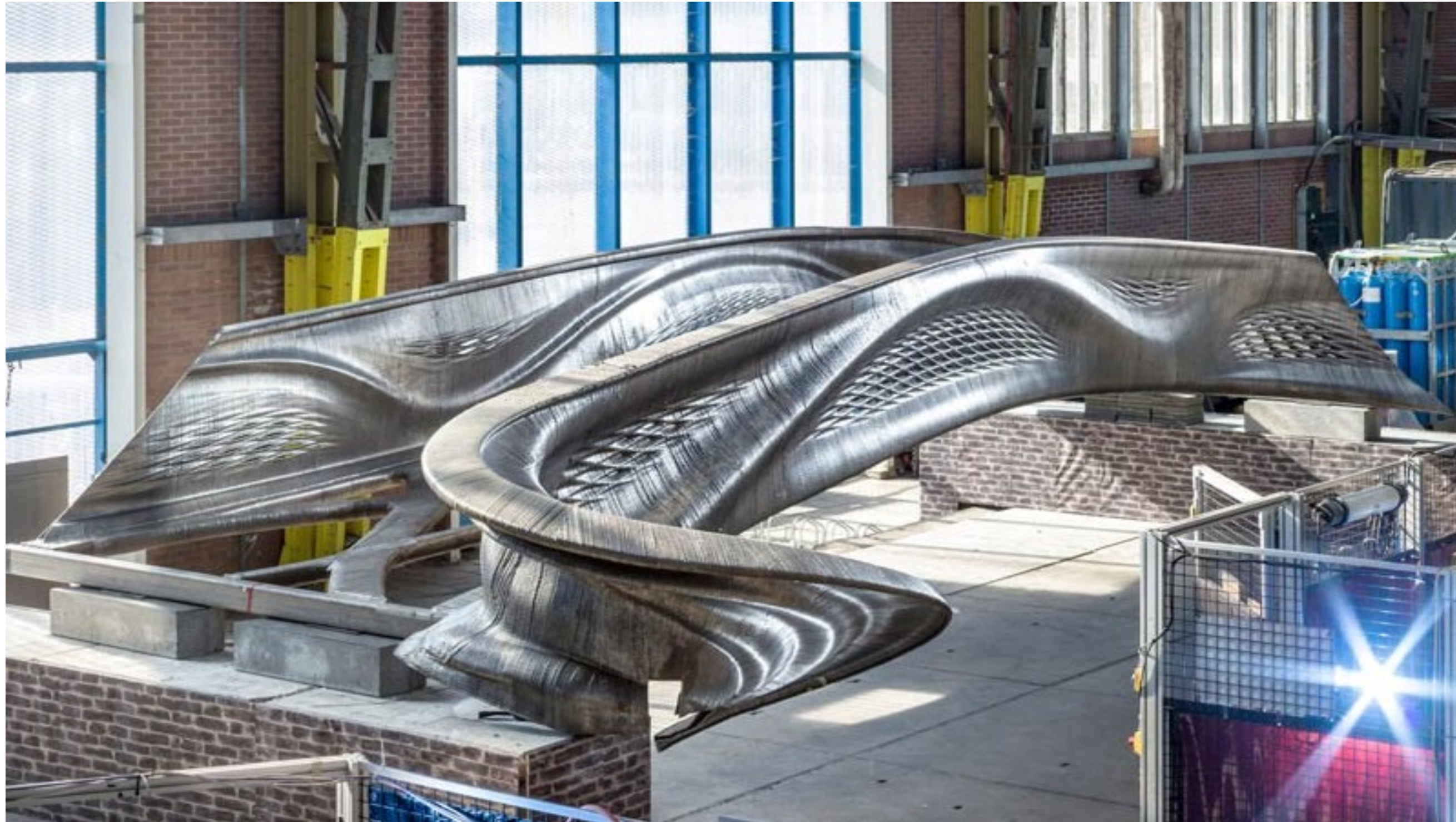
3D printed steel bridge
