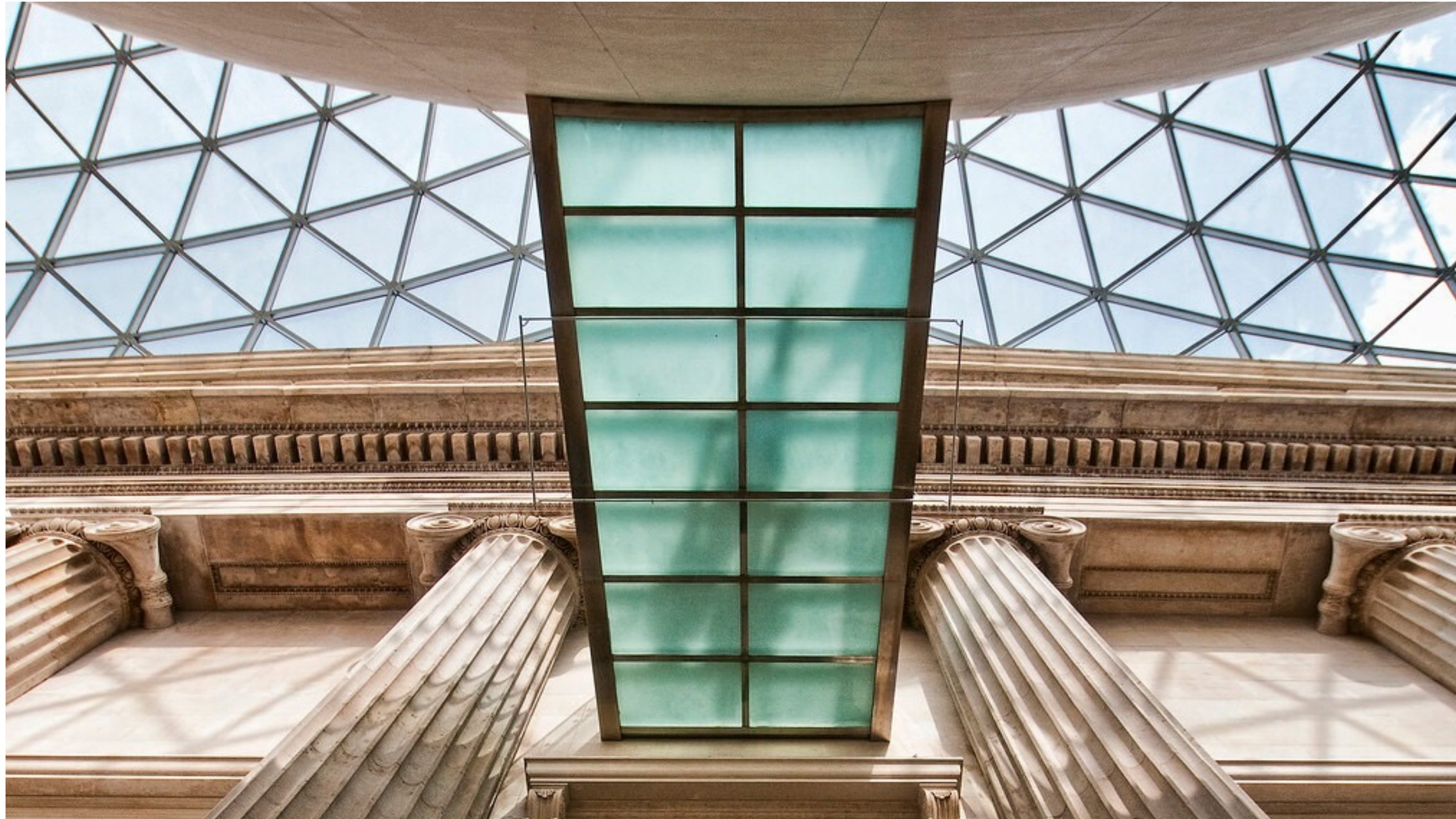
Bridge connecting the atrium and gallery spaces - The british museum
