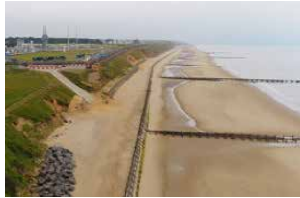
Figure 1 (left). The cliff coast at Bacton Terminal showing small-scale protection works. (Photo by Royal HaskoningDHV)
