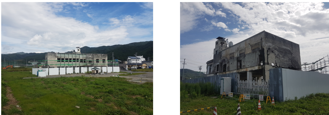
Figure 1.1: Destroyed Government building in Otsuchi Town during the 2011 Tohoku Earthquake Tsunami [pictures: J.J. Roubos]
