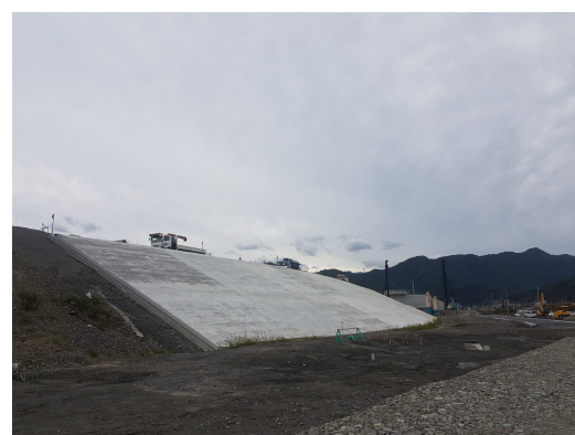
(b) Sea dyke under construction, height = 14.6m
