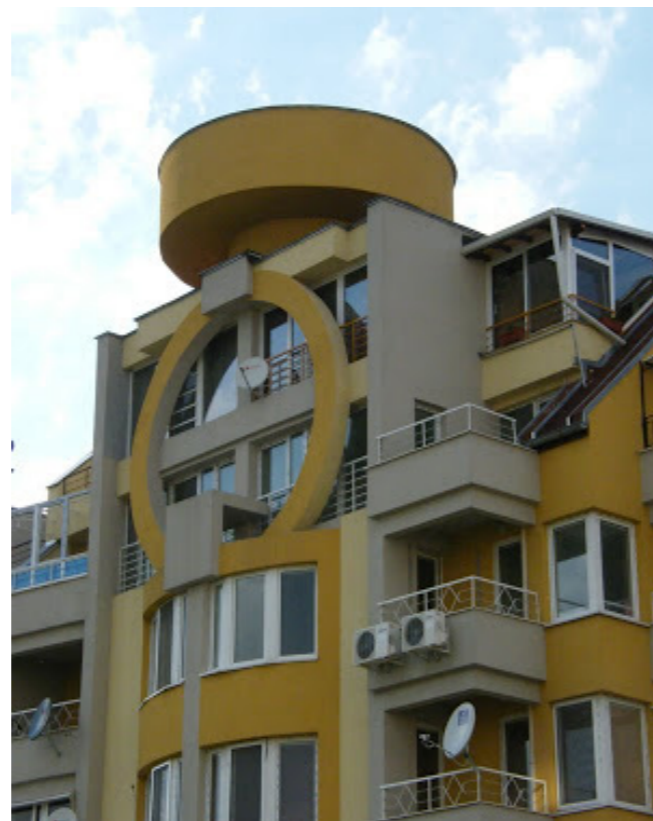
fig. 20 Residential Building, Sofia
