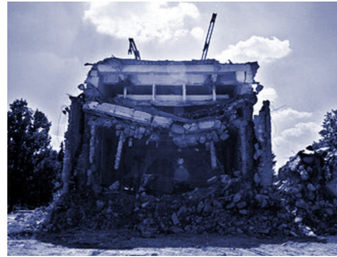
fig.10 Demolition of the Georgi Dimitrov Mausoleum, Sofia
