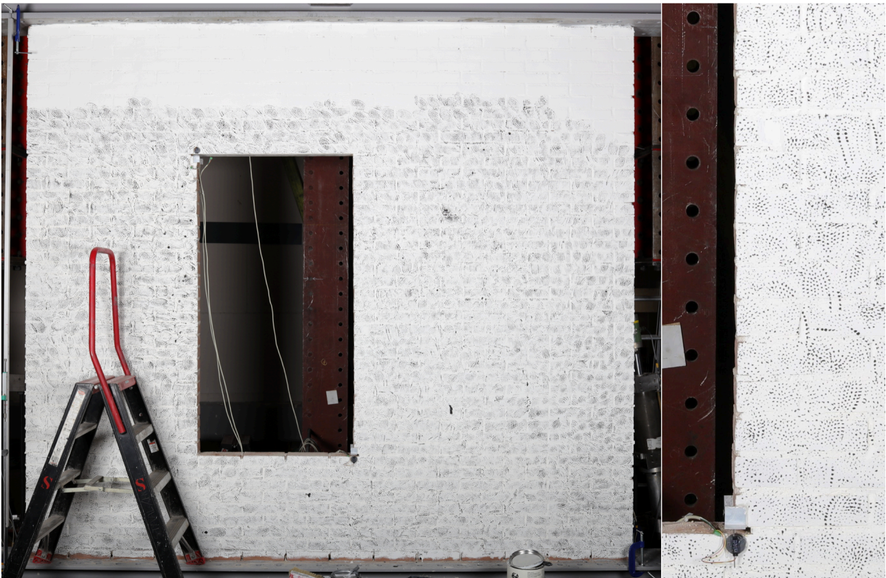
Figure 2.9. Patterns being applied to the wall.
