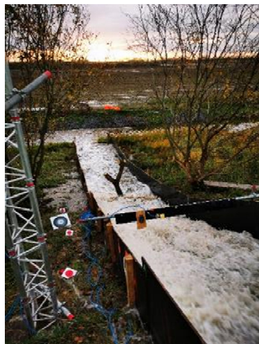
Figure 4. Anomaly test section with a tree trunk at the toe of the dike.
