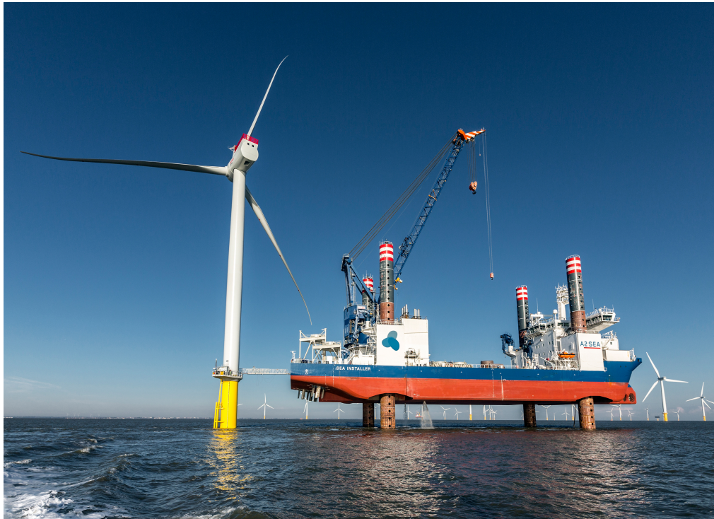
Figure 1.3: Offshore wind turbine maintenance with a jack-up vessel
