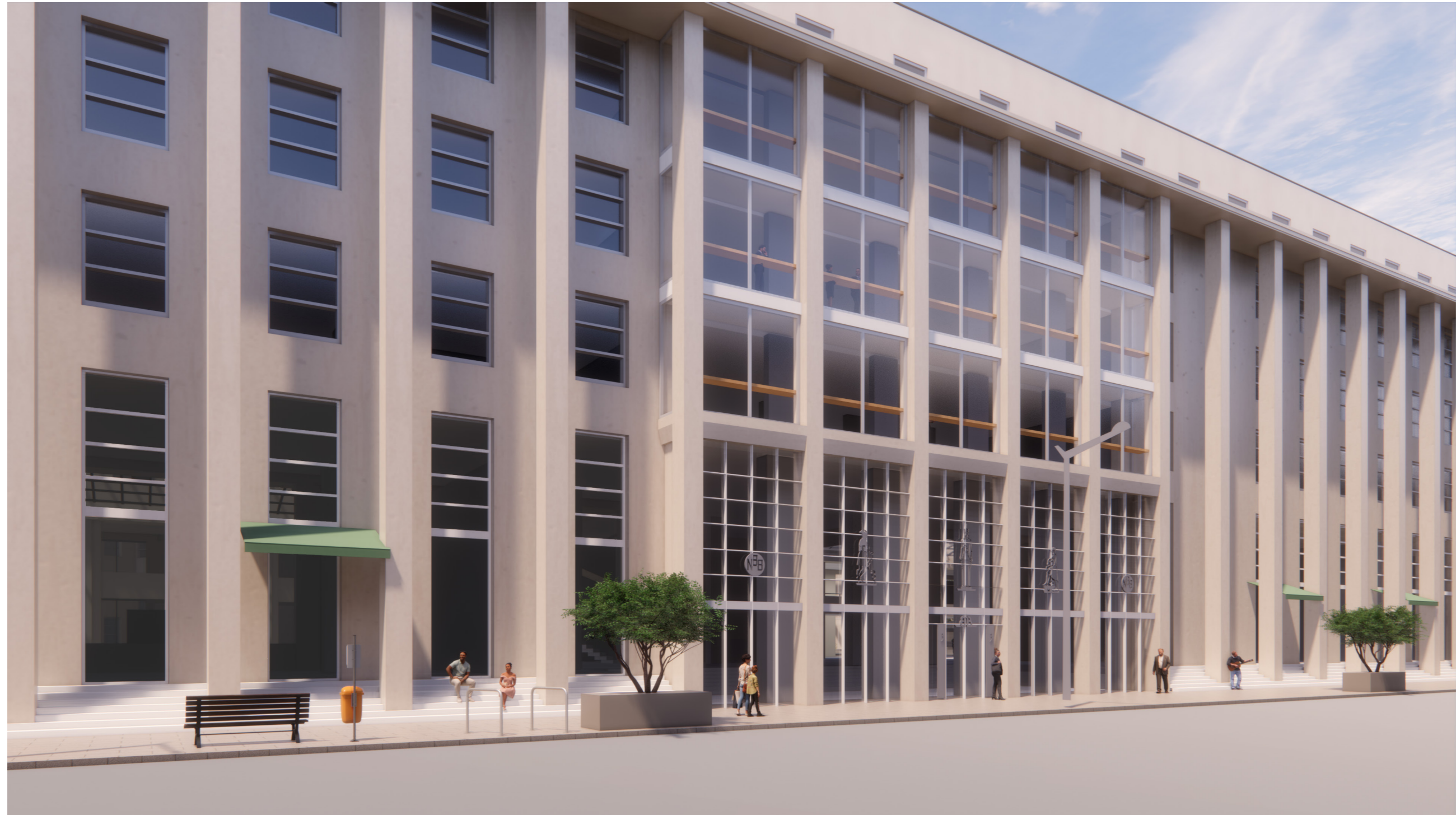
New window frames showing the employees of the bank
