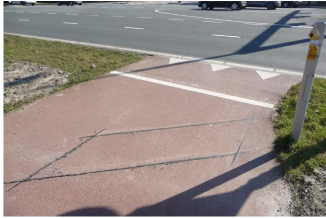
Figure 3: A loop sensor (Dirk de Baan, n.d.)
