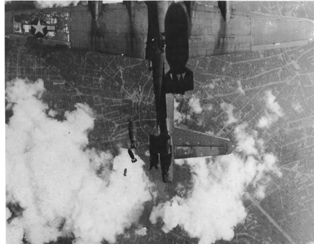
(b) Photograph 1 showing stabilizer after bomb impact.
