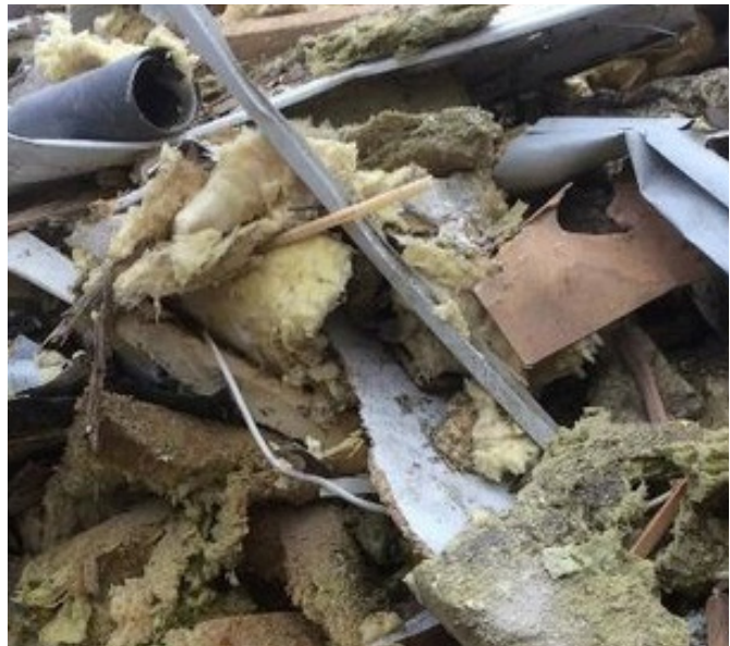
Demolition waste including mineral wool. Credit: Juho Yliniemi et al., 2019
