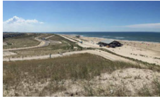
FIG. 4.26 The coast of Petten after sandy reinforcement (2018), including a new 60 m-wide dune system. Source: J. van Bergen.
