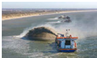
FIG. 2.7 Shoreface nourishment in North Holland, NL 2020 (middle). Source: Rijkswaterstaat.
