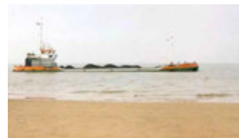
FIG. 2.8 Channel wall nourishment by hopper dredger 2011 (right). Source: Rijkswaterstaat / Deon Slagter WG 2011.
