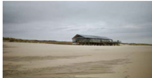
FIG. 3.29 Right: photo of the beach pavilion 'the Coast', on the left the extended deposition tail of the elevated pavilion is visible, heightening the beach and foredunes. Photo: S. Veldhuisen (2023).
