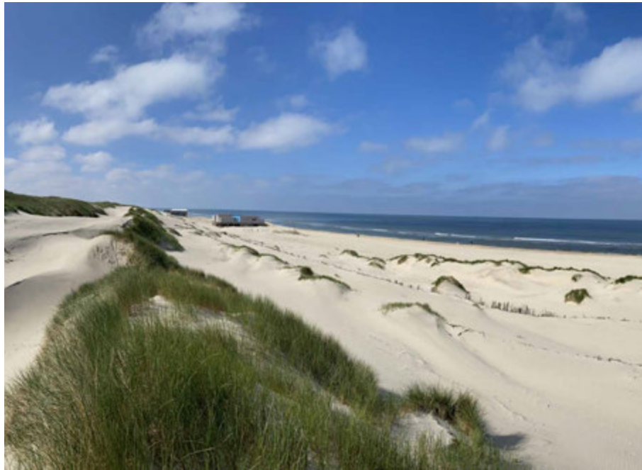
FIG. 3.51 (+ sections in Figure 3.47): Buried fences (right) at Camperduin (2021) providing a substantial seaward extension of the dunes ( > 250 \text{ m}^3/5 \text{ y} ), combined with vegetated foredunes (middle, left) and embryonal dunes (right). Image by the author.
