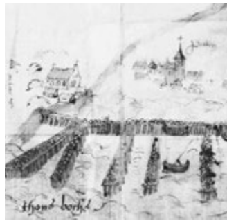
b) The village of Petten around 1552 by Jan van Scorel, with pole construction as the last sea defence.
