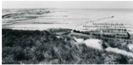
Traditional planting of Marram grass and sand screens near Cadzand, around 1900. This old BwN technique could be re-employed in the creation of safe grounds for urban beach development.
