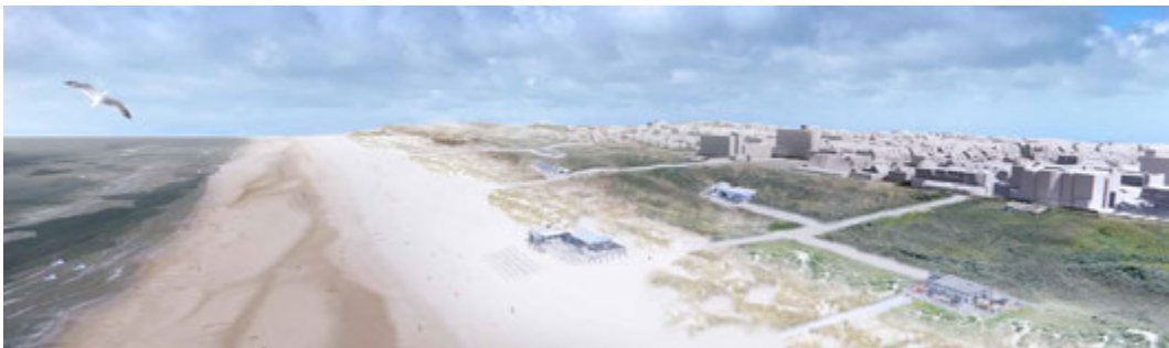
d) Noordwijk as a Sand buffer phase 3 reinforcement, promoting BwN-based, terraced dune widening
