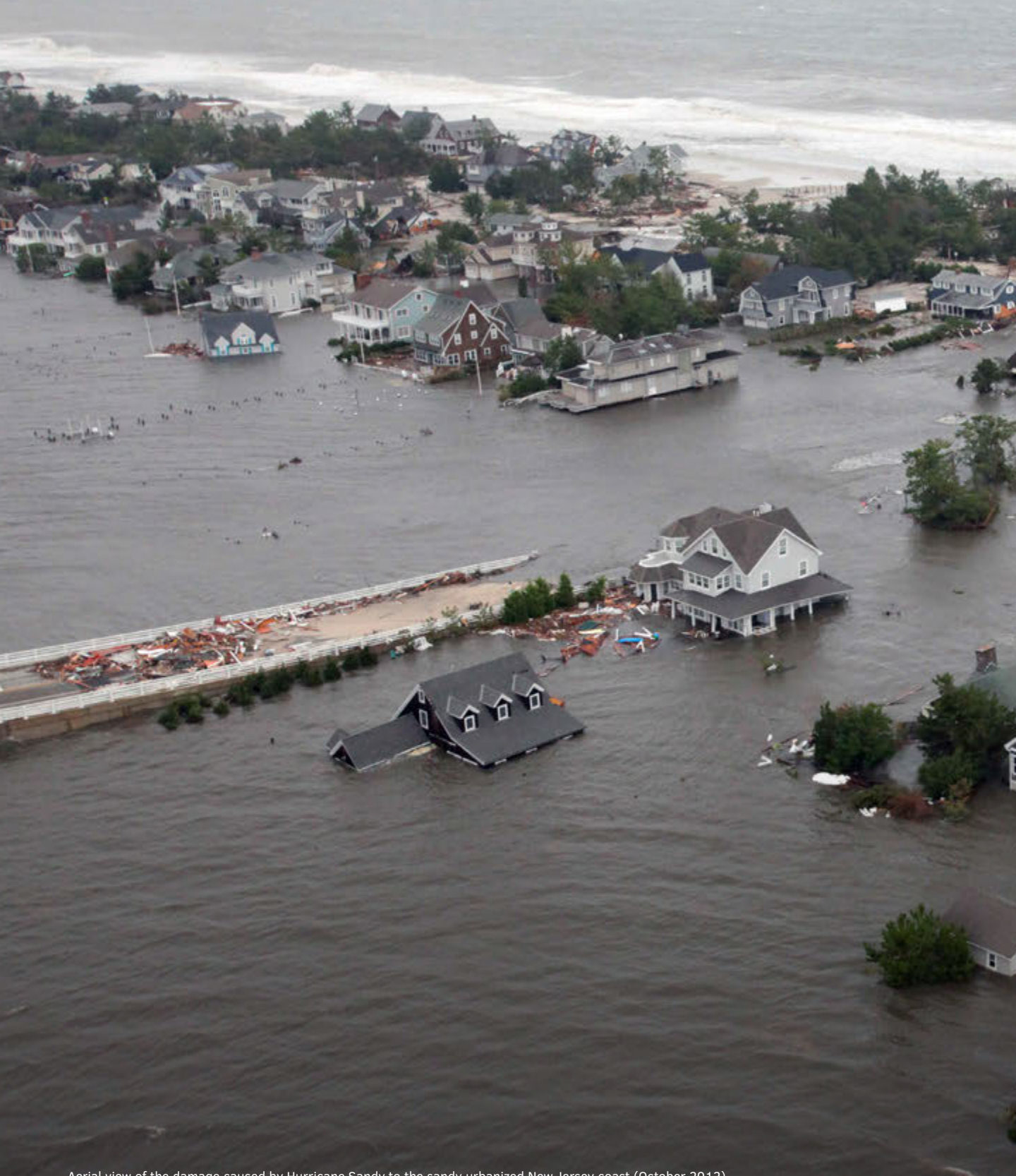
Aerial view of the damage caused by Hurricane Sandy to the sandy urbanized New Jersey coast (October 2012). Source: National Guard of the United States.
