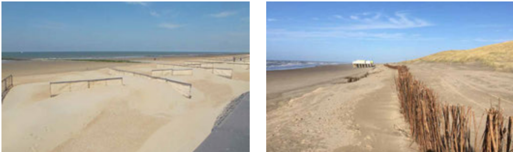
FIG. 3.49 Example of artificial fencing in a cross-formation on the Belgian coast to prevent sediment from blowing onto the boulevard (left) and natural brushwood screens at Petten (right). Images by J. van Bergen.
