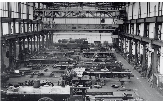
Fig. 6 The Lochal when it was still a locomotive repair shop (Mecanoo, n.d.).
