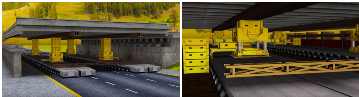
(A) Placement of new bridge with SPMT.
