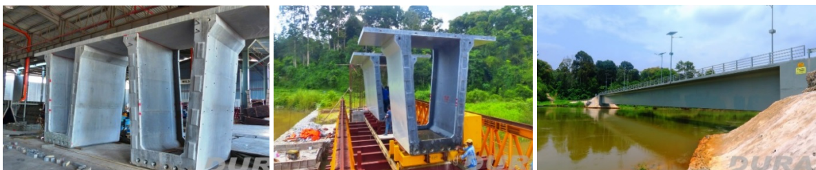
(a) Prefabricated UHPC bridge elements.
