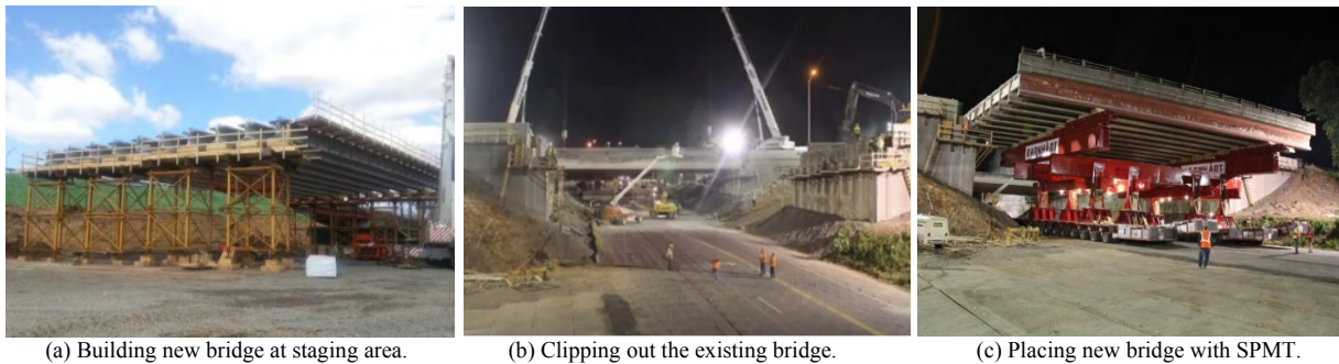
Fig. 4. Replacement of the two I-84 bridges over Marion Avenue (Atkinson, 2015).
