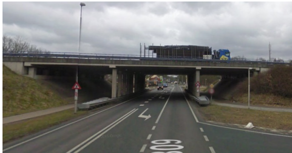
(a) Existing three span plate bridge in A28/N309.
