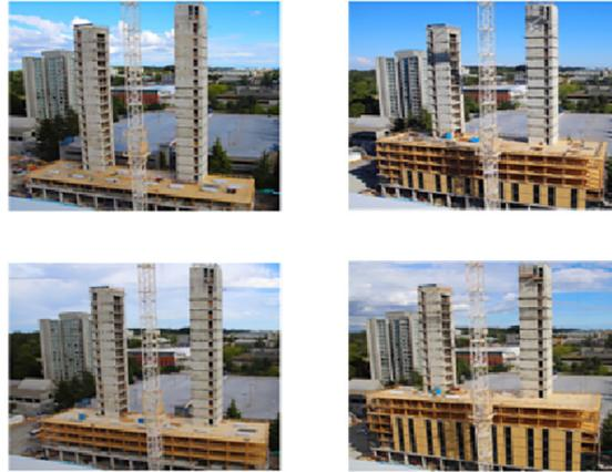
Figure 2.4. *Construction sequence of mass timber elements brock commons[9]*
