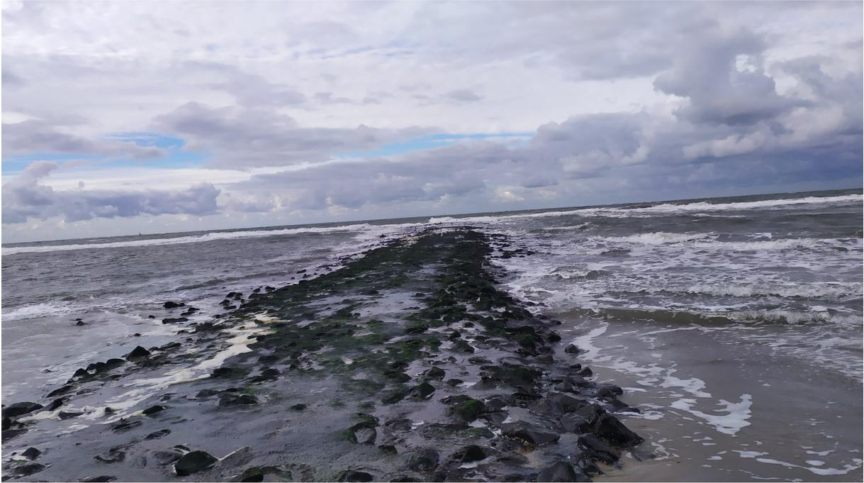
Figure A.4: Cross-shore groyne during low water. It consists mainly of rocks and tar.
