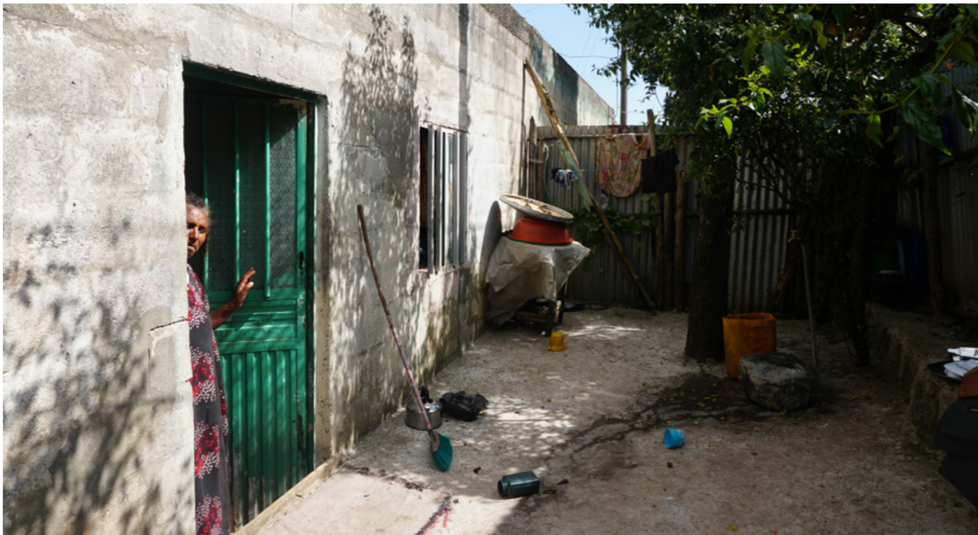
Governmental housing in Kolfe built from concrete blocks
