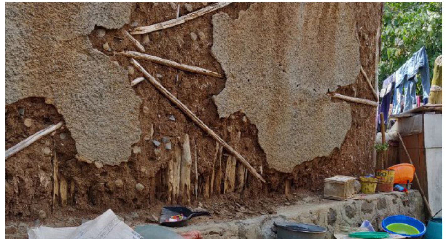
Informal housing walls made from chicka, stones and wooden frames in Kechene
