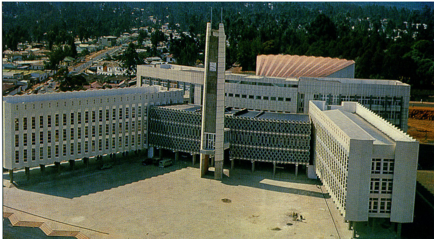
City Hall of Addis Ababa, 1964
