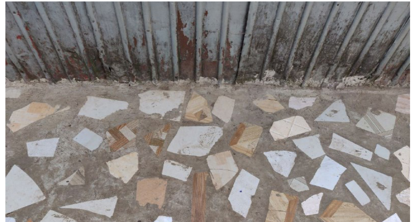
Broken tiles used in concrete for pavement in Kechene
