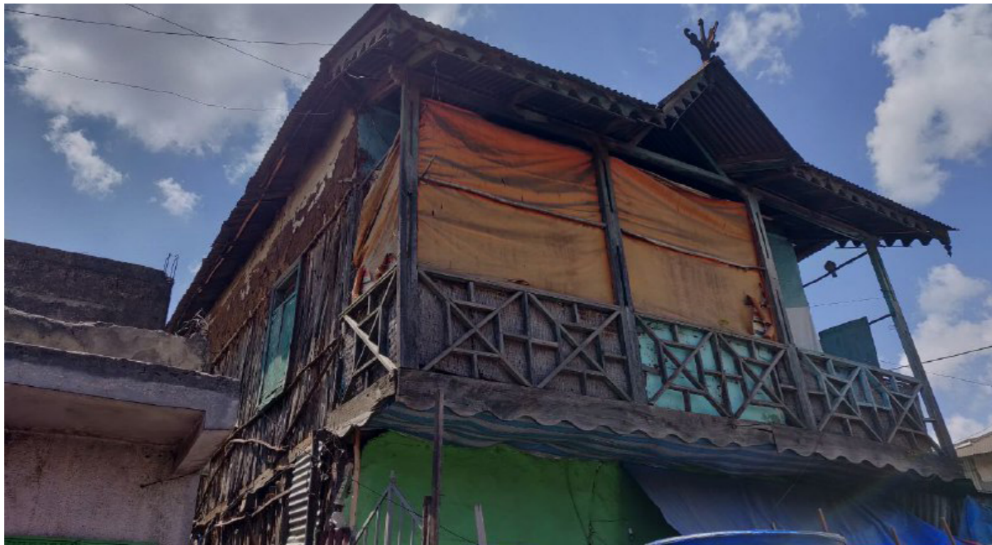
Historical buildings transformed into informal housing, Tallian, Addis Ababa
