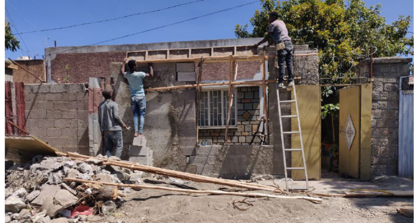
Construction of a new shop in Gerji
