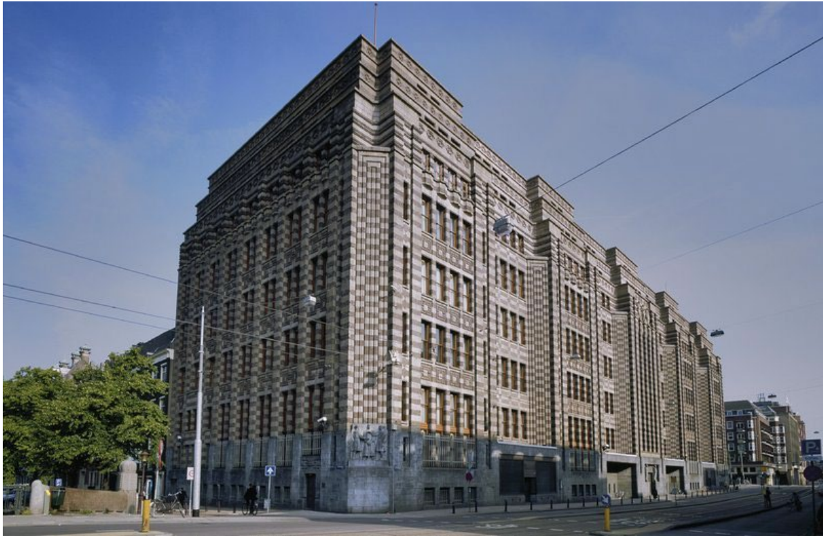
Figure 7. Headquarters for the Dutch Trading Company (NHM: Nederlandse Handels-Maatschappij), Vijzelstraat in Amsterdam, by K.P.C. de Bazel (1926). Today, the building has been renamed De Bazel and is used by Stadsarchief Amsterdam.
