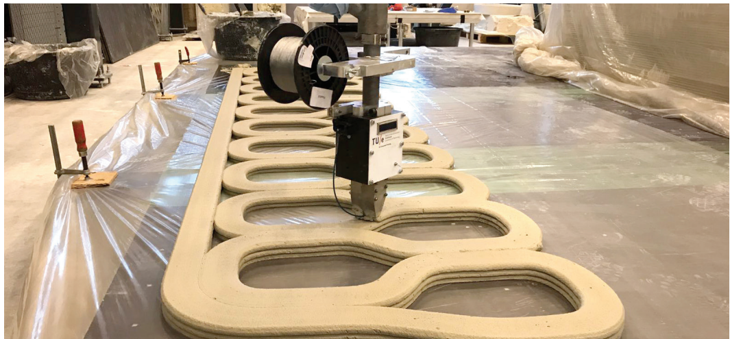
FIGURE 5 3D printing concrete with a directly entrained reinforcement cable.
