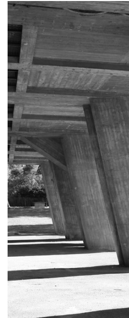
Unite d'habitation View of pilotis
