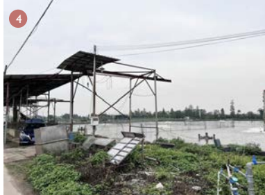
4 Cable setting in the fish pond
