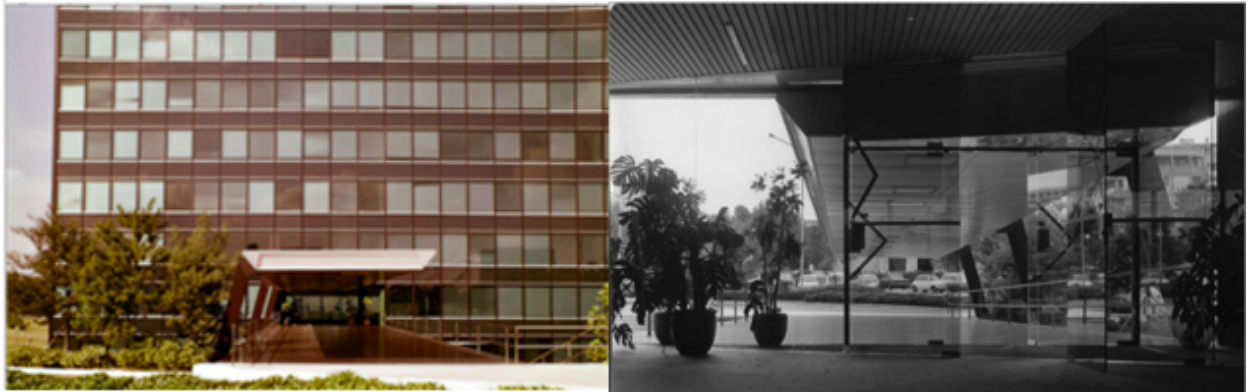
Figure 20. ENI Palace main entrance from the outside and inside.
