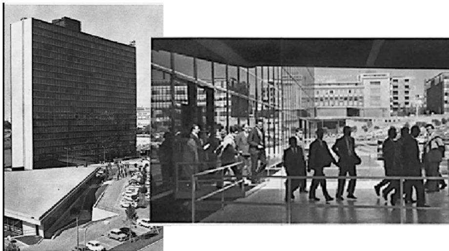
Figure 21. ENI Palace at EUR and the canteen building.
