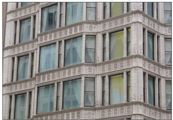
Figure 7: the Reliance building with a characteristic Chicago window, optimized for letting in daylight 6
