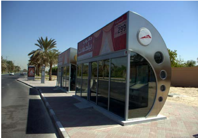
Air Conditioned bus stops
