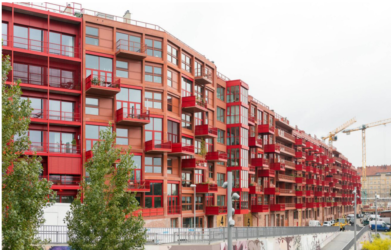
Figure 39: Street front of the Lokdepot
