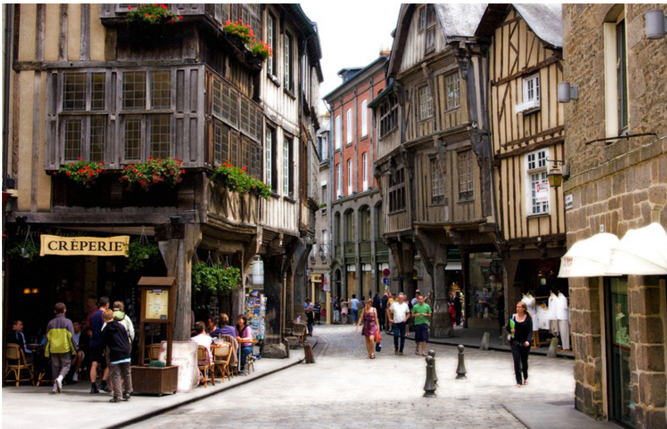
Figure 30: Dinan, France. Active groundfloors and narrow streets make places seem more lively
