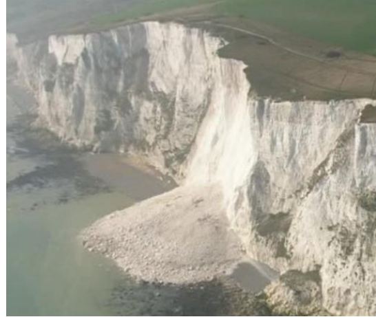
Figure 1: example of coastal chalk cliff collapse (picture by BBC)
