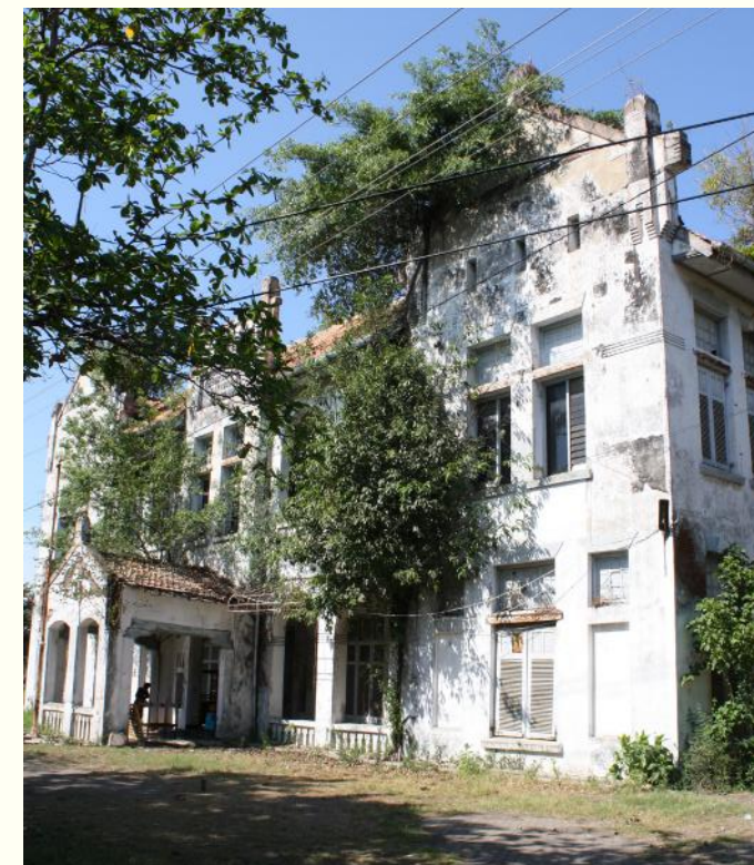
UPTOWN JAVAHOUT BUILDING
