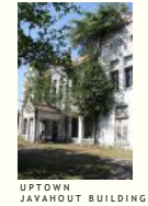
UPTOWN JAVAHOUT BUILDING
