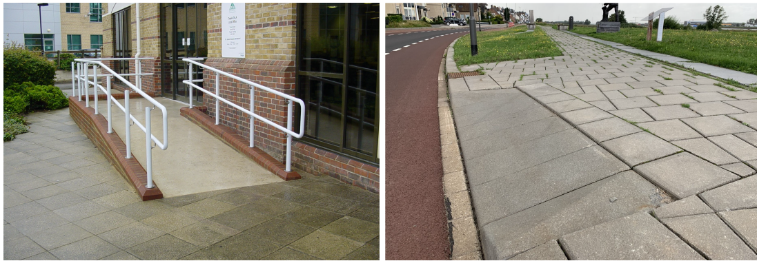
(a) A ramp in front of a public building [36]. (b) A curb ramp providing access to the sidewalk [37].
