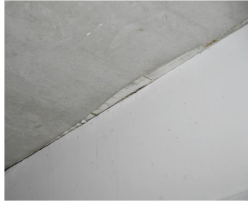
Figure 5.34 Gradual walking of elastomeric bearing pads (Adviesbureau Hageman).
