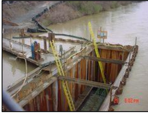
FIGURE 7.11: DRY CONSTRUCTION SITE
