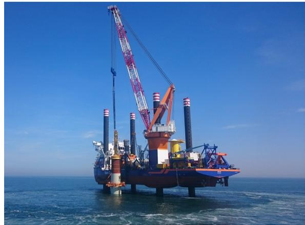
(b) Jack-Up Barge Aeolus, Van Oord, installing a Monopile[37]
