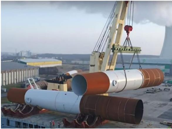
(a) Transfer of an MP using a spreader bar for the Walney Extension wind farm (Dong Energy)[13]
