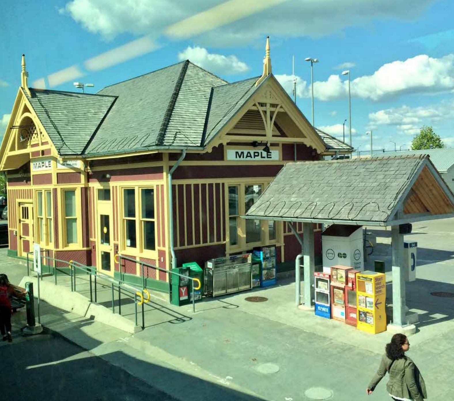
Figure 16 Maple Newmarket GO Historic Station. Source: Photography by Sean Marshall
