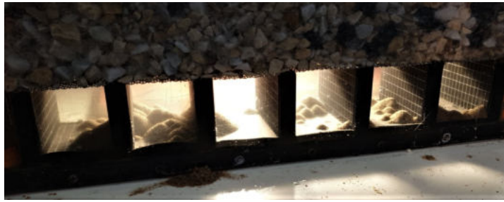
Figure 5.16: Heaps of sand inside the sand trap, which are due to channelling in the granular filter layer
