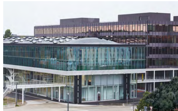
Fig. 1 – Case study building, South-West facade
