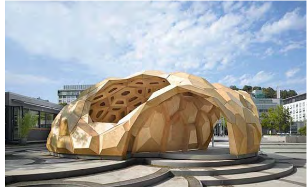
ICD-ITKE Research Pavilion 2011. ICD-ITKE University of Stuttgart. Photo by Roland Halbe.
