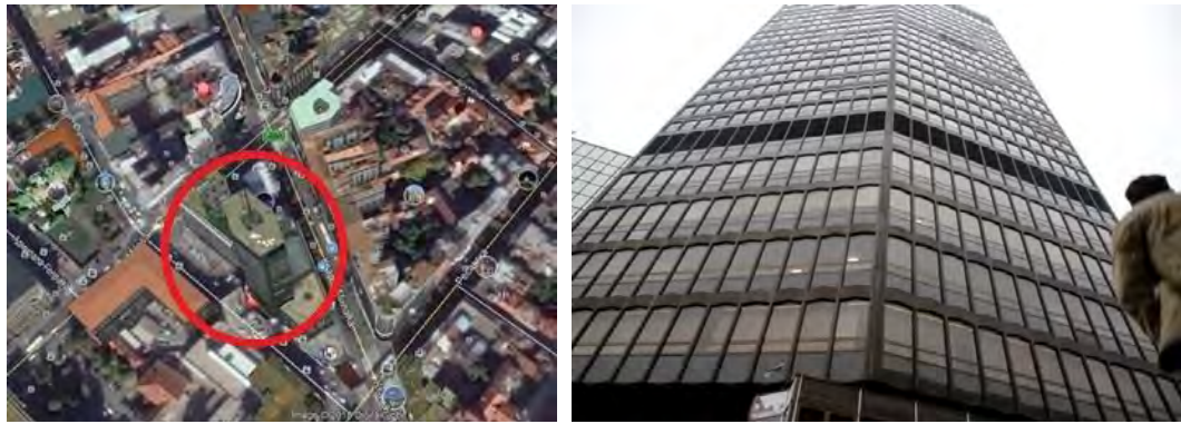
Figure 5 - "Beogradjanka" office building, Case Study I
