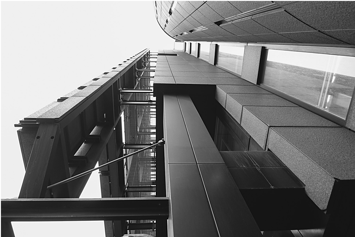
FIGURE 5.6. 100 Liverpool Street at the entrance to Broadgate Circus, designed by Arup Associates under Peter Foggo (1985–1987); note the thin layer of detached stone cladding. © Danielle Willkens, 2013.
