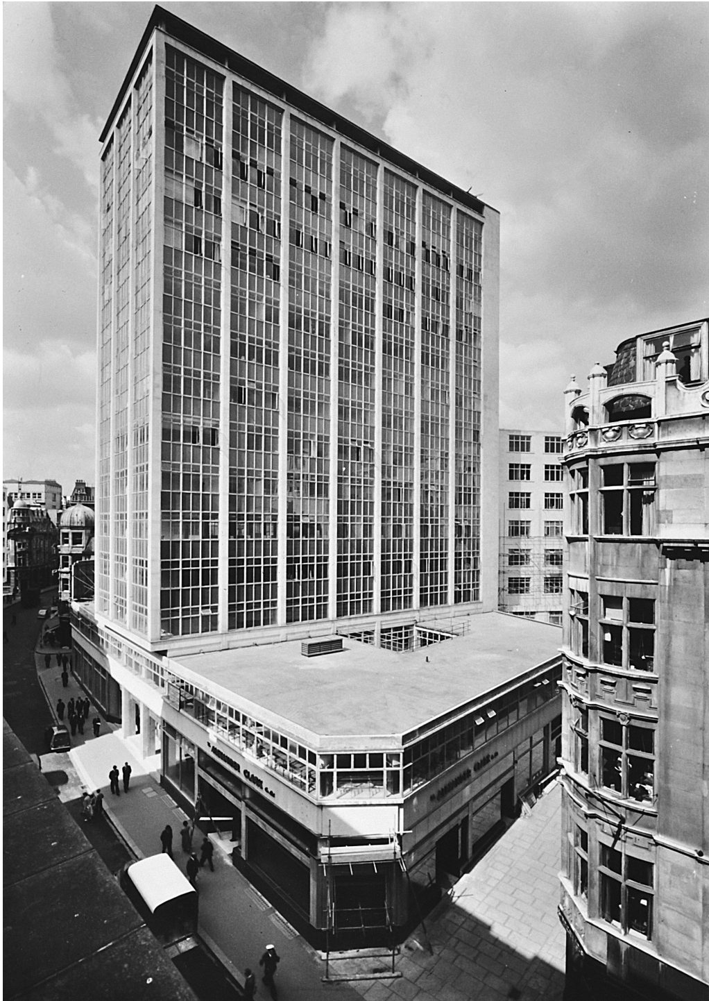
FIGURE 5.2. Fountain House, designed by W. H. Rogers, 1957, for the City of London Real Property Company.
