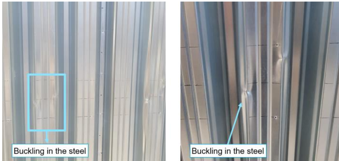
Figure 36 Buckling in the steel sheet after testing at load locations.
