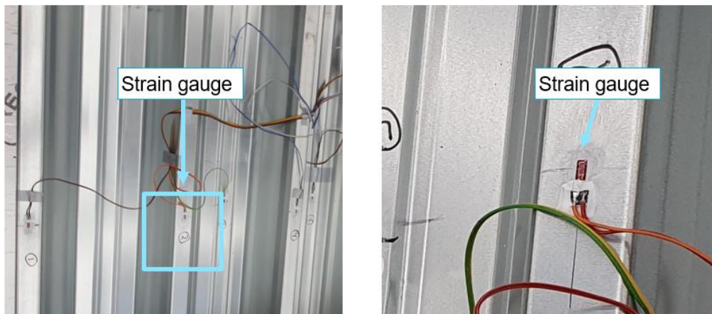
Figure 26 Strain gauge on the steel sheet.
