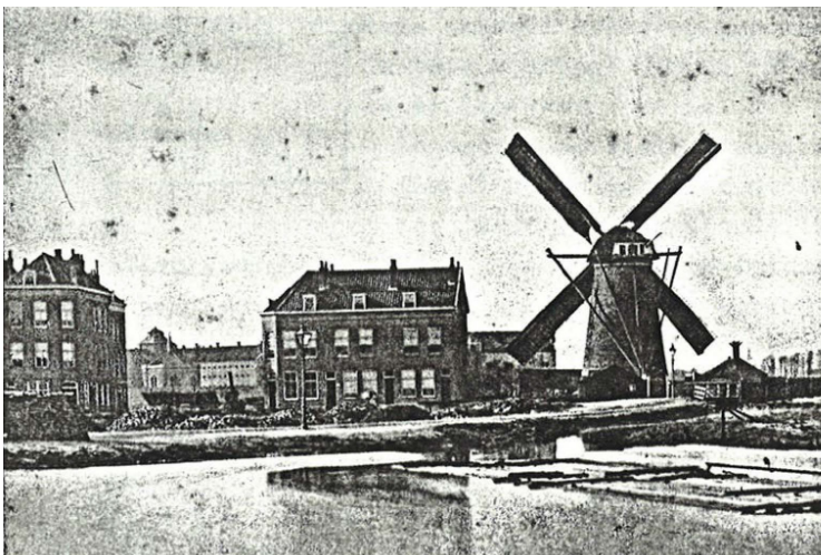
'Bloomersdijk windmill' 1875 (Rotterdam Municipal Archives) Seen along the Rotte in the industrial section near current day Noordplein. Shortly after this photo is taken the windmill will be demolished and replaced with a steam powered pump.
