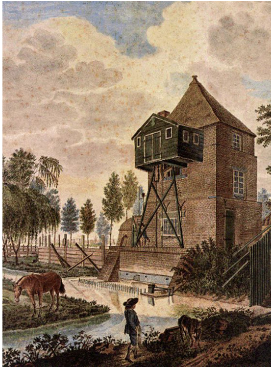
'The steam pumping station of the Blijdorp polder' ca 1820; J.Z.S Prey (republished in: K. van der Pols & J .A. Verbruggen "Steam drainage in the Netherlands 1770–1870" 1996)
