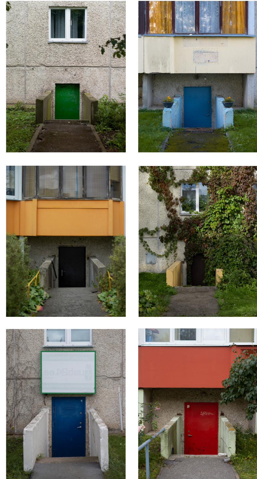
[figure 7] Closed Basement Spaces and Failed Basement Shops
