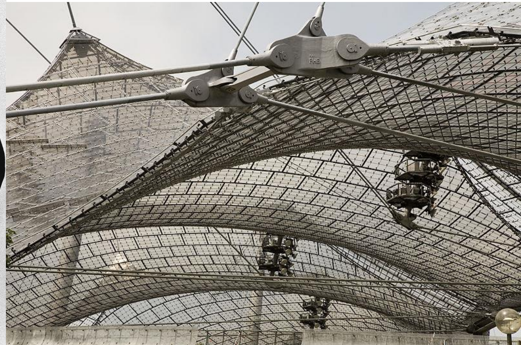
Frei Otto – Munich Olympic Stadium
