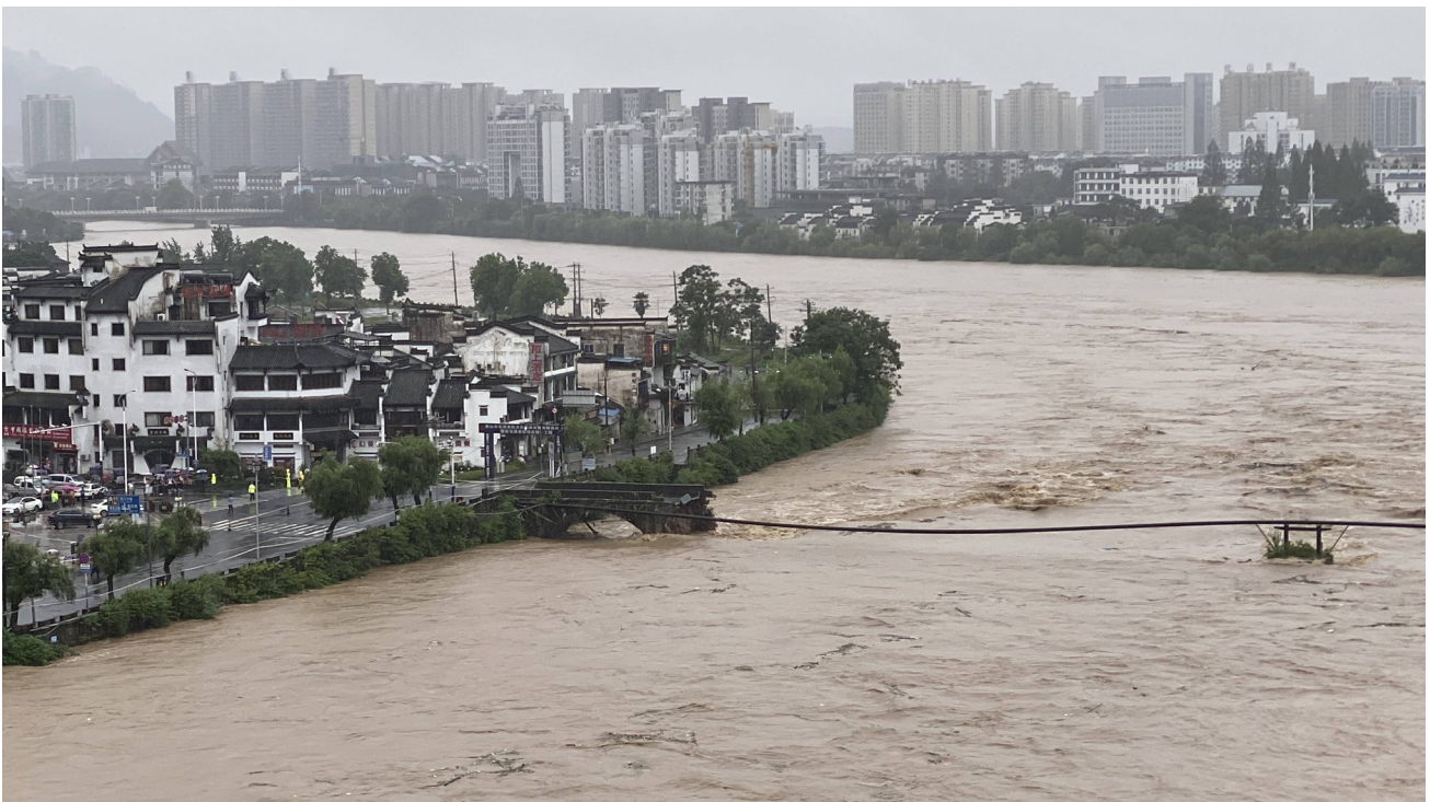
Flood destroys ancient bridge in east China, a photo taken on July 7, 2020 Source: http://www.xinhuanet.com/english/2020-07/07/c_139194709_2.htm
