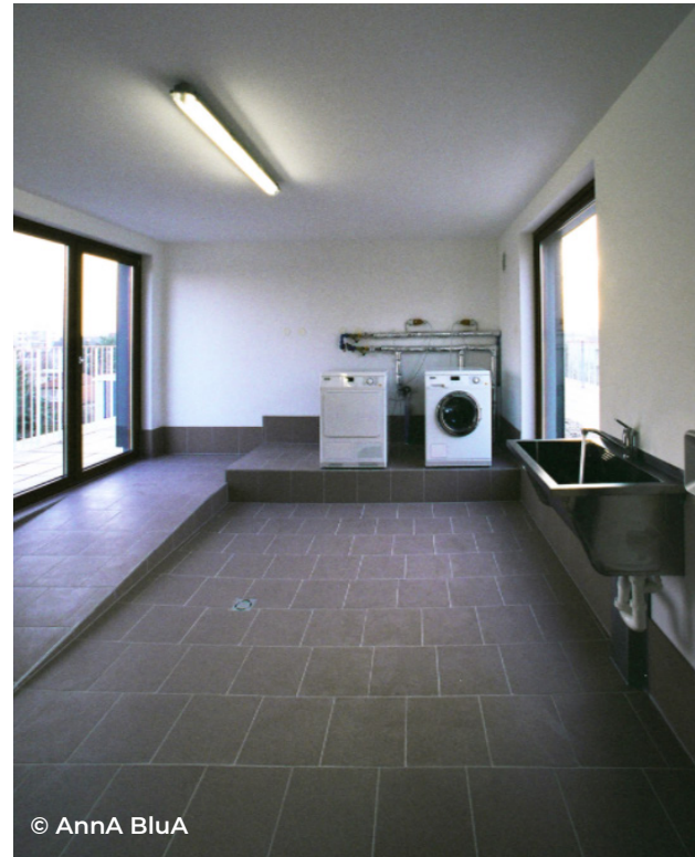
Inside the laundry room
