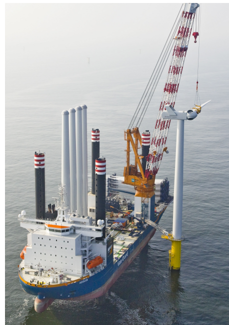
Figure 1.1: Blade installation by the Aeolus
