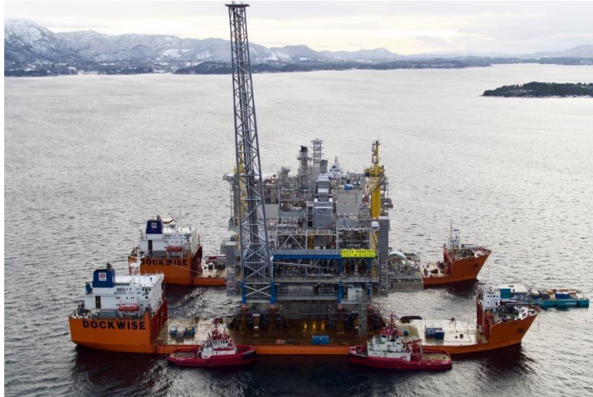
Figure 2-6 Twin barge float-over (Ace winches, 2023)
