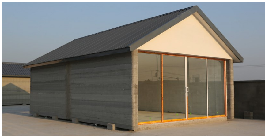
FIGURE 2 3D printed concrete house
