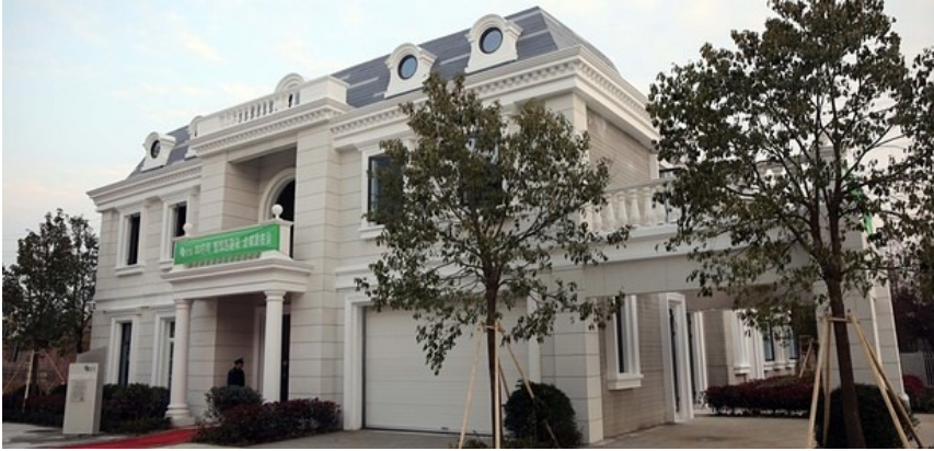
FIGURE 3 3D printed concrete villa
