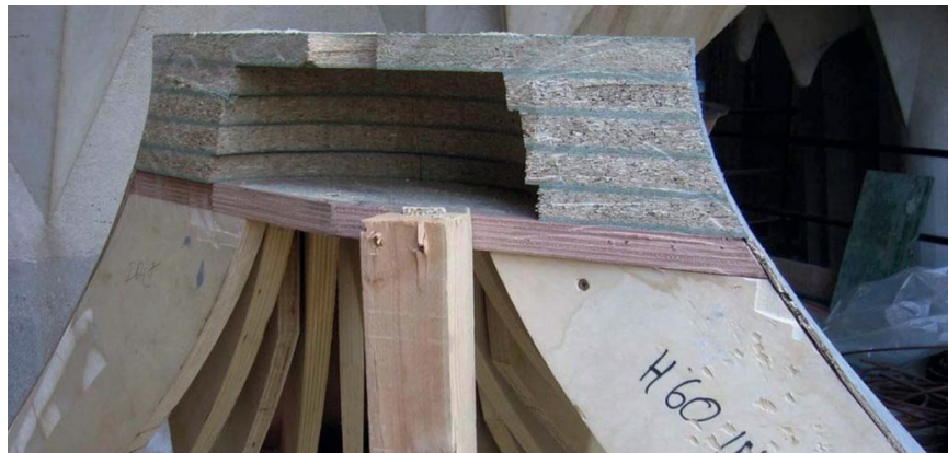
FIGURE 8 Wooden formwork for Sagrada church (Espel, Gómez-Serrano, Grima, Burry, & Aguado, 2009, p. 108)
