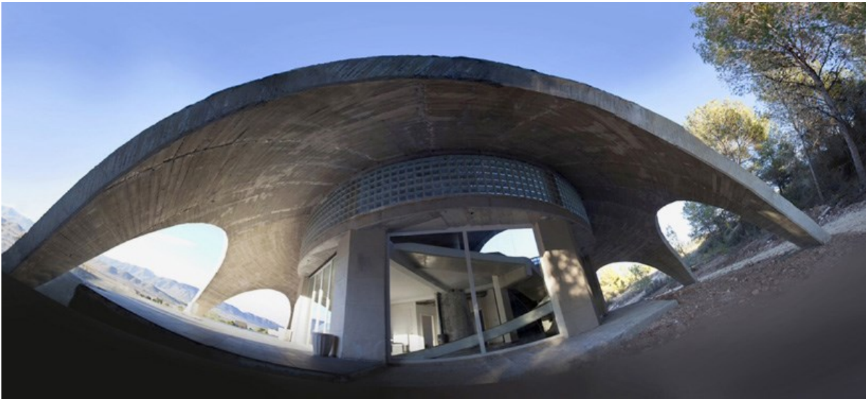
FIGURE 10 Claudio Hebberecht - freeform concrete dome
