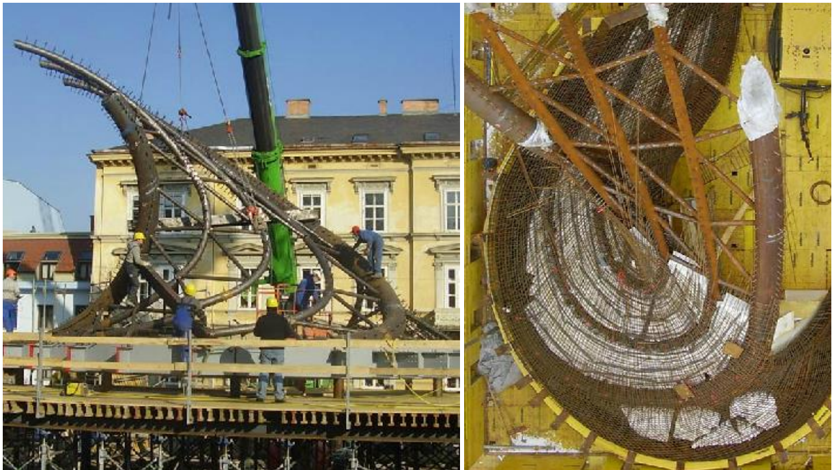
FIGURE A. 19 STAIR STEEL STRUCTURE (CONVEX, 2008)
