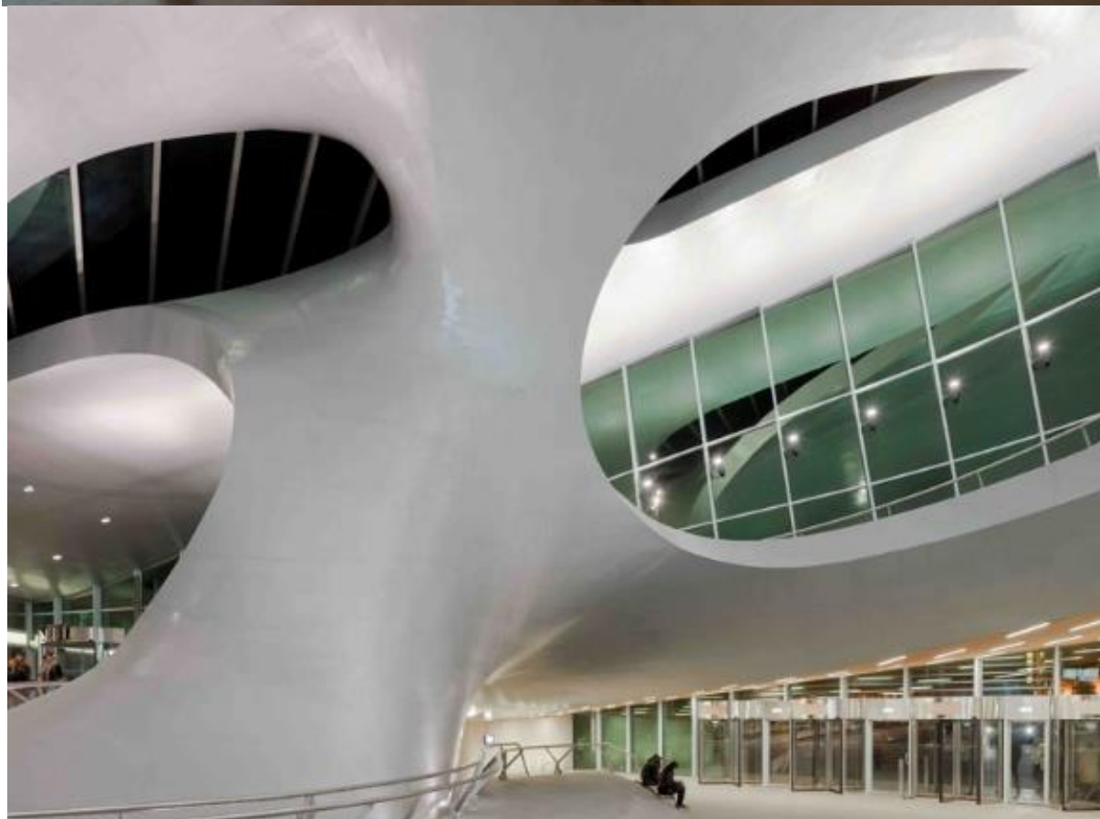
FIGURE A. 23 ARNHEM STATION – STEEL STRUCTURAL COMPONENTS (DESIGNALMIC, N.D.)
