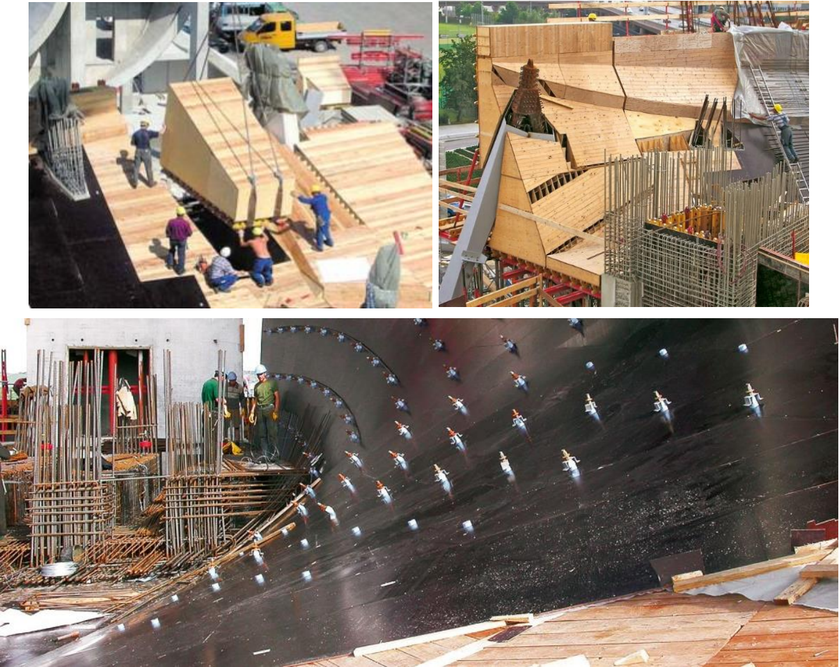
FIGURE A. 17 MERCEDES-BENZ MUSEUM BUILDING CONSTRUCTION (PERI, 2006)
