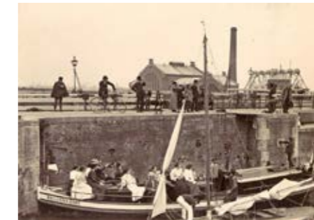
King Willem III laid the first stone on April 29, 1870. Five years ago, work had been done with a lot of setbacks on the construction of the cofferdam that formed the largest part of the closure. On 25 September 1872 the first ship sailed through the lock.
