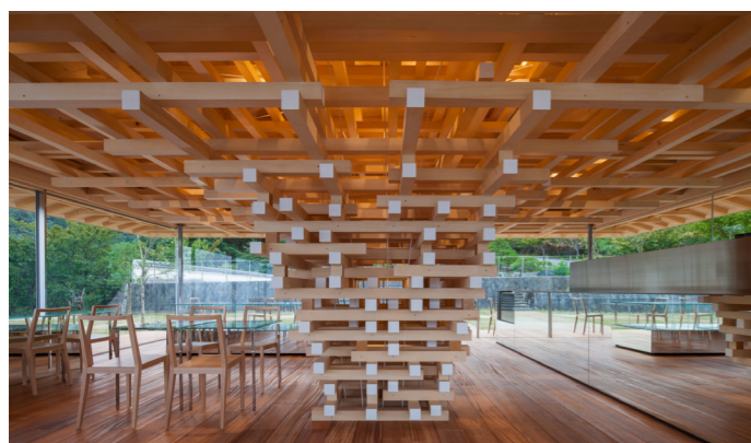
Figure 6.6: Coeda house tree-like structure (Kawasumi-Kobayashi Kenji Photograph Office, n.d.)
