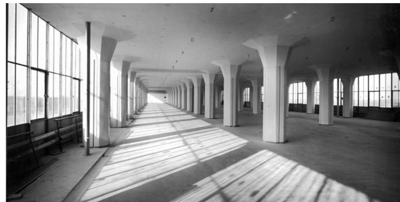
Figure 6.17: Mushroom columns in de Van Nelle factory (Tjasker, n.d.)
