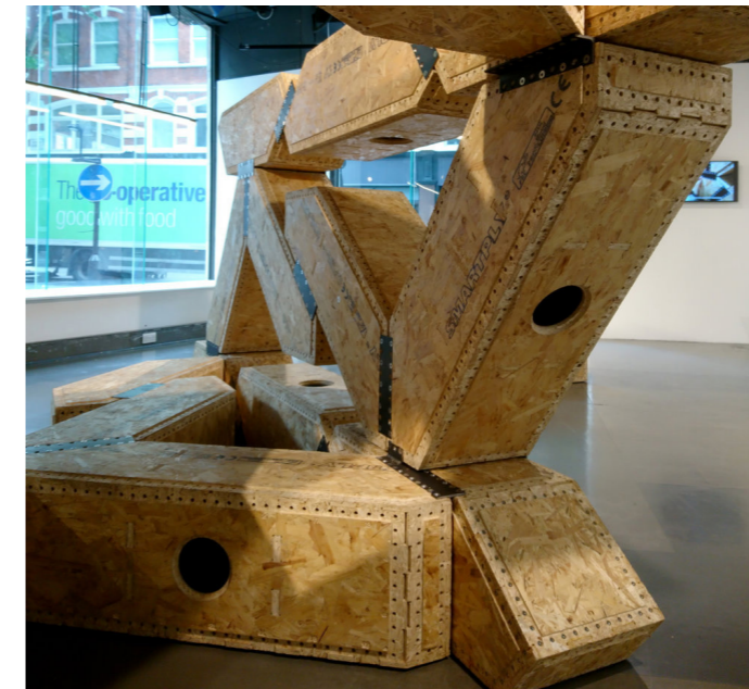
Figure 6.2: Hollow OSB blocks (I. Tedbury, 2018)
