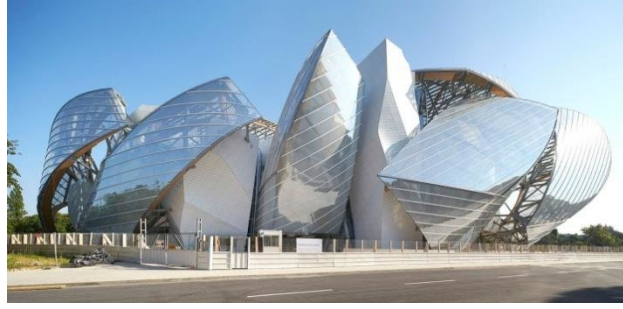
Figure 3.3: Louis Vuitton Foundation - double side bent glass panels for canopies
