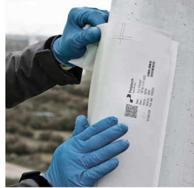
(b) Application of a premolded leading-edge protection shield; photograph reproduced from Polytech (2023).
